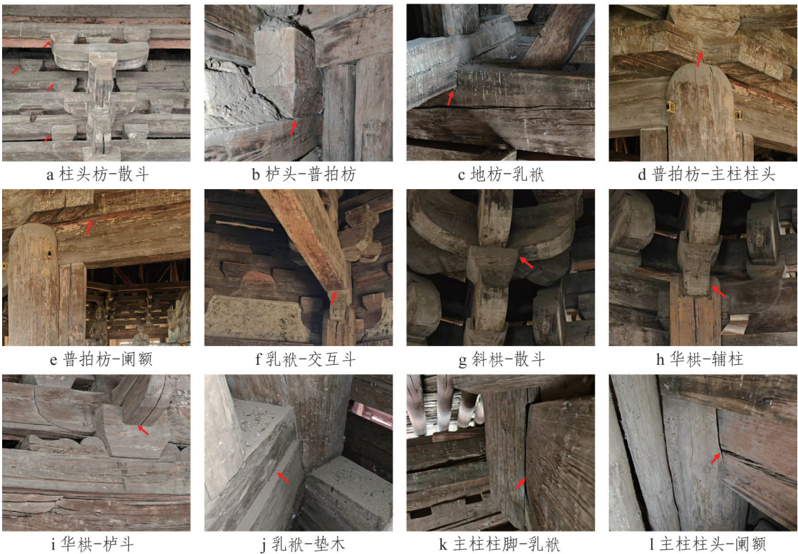
图7 典型弦-弦连接界面木构件组合 Fig.7 Typical timber component combinations with the tangential-tangential contact interface
